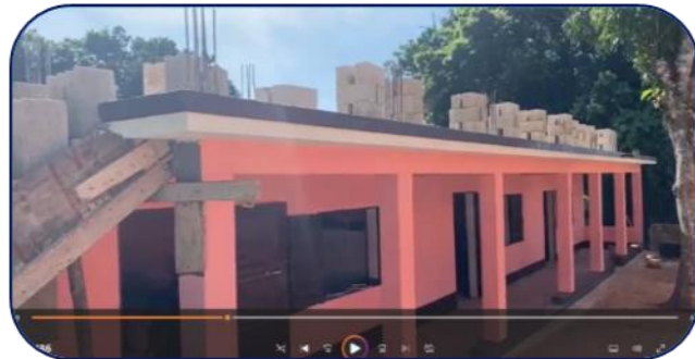
Above: 1 st floor complete – Dec 2023
