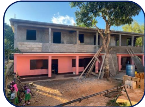
Above: 2 nd floor nearly done – Jan 2024
