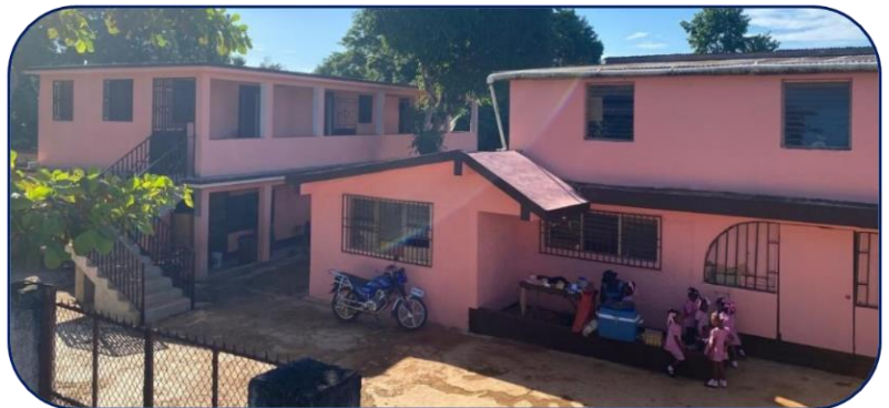
Mussotte Elementary. The expanded annex is on the left.
