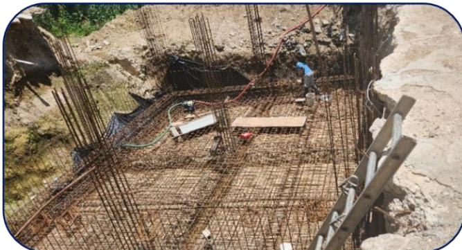
Left: Cistern under construction.
