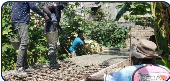
Left: Culvert being built.
